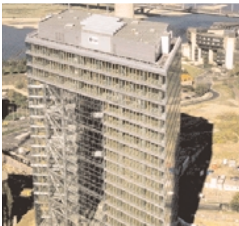
The Stadttor in Düsseldorf, one of many famous constructions equipped with Paroll double-floor systems.
