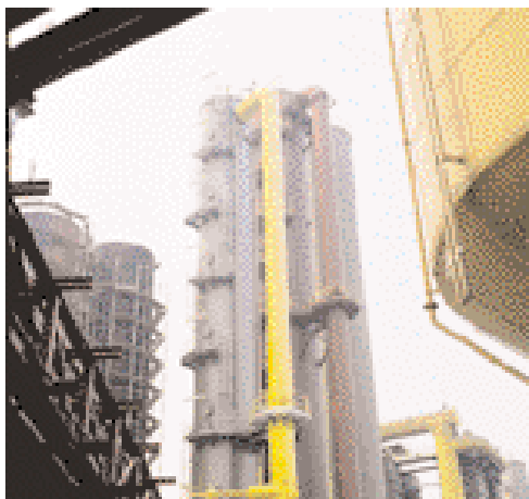
The Steiner group is focussing on technology for the chemical and petrochemical industries and components for the iron and steel industry.
